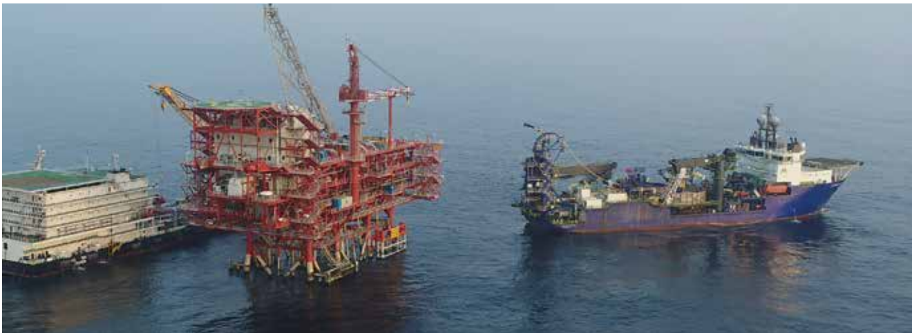
CRP modifications underway
