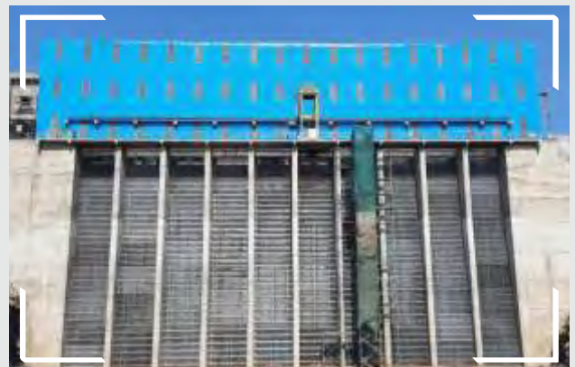
Kundalia Lift Irrigation Package, M.P. India Trash Rack Grab Cleaner Mechanism 31 m height and 4.5 m width ( Per bay width). Total no of bay is 10 - 3 nos.
