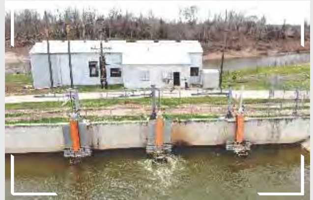
GCWA Pump House Levee Structure, Sienna Parkway, TX, USA Knife Gate Valve Dia. 72" - 3 nos.
