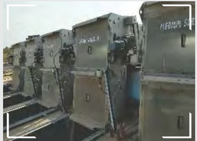
90 MLD STP Bellendur, BWSSB, Bengaluru, India
