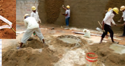
Work in progress at Bengaluru project site
