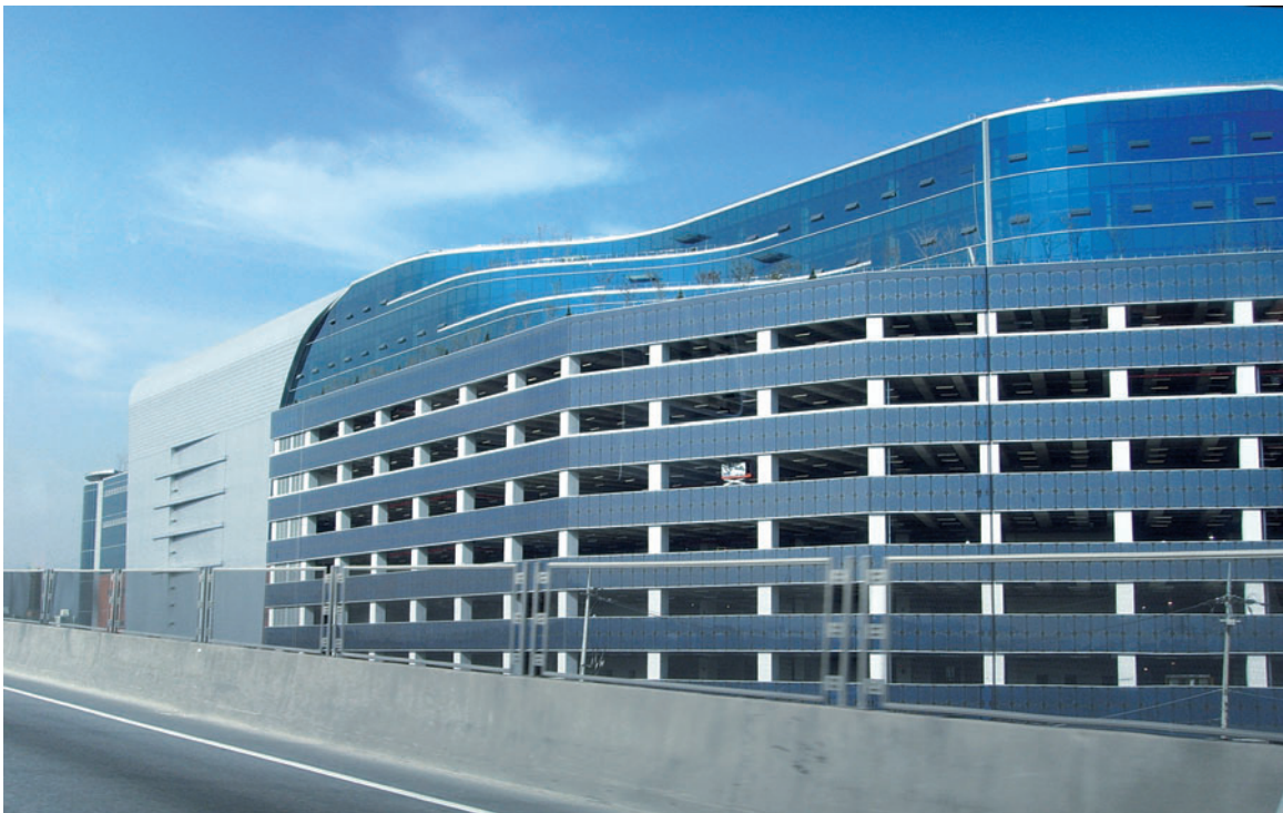
DongNam - currently largest building-integrated photovoltaics system in South Korea with a total capacity of 607.5 kWp
