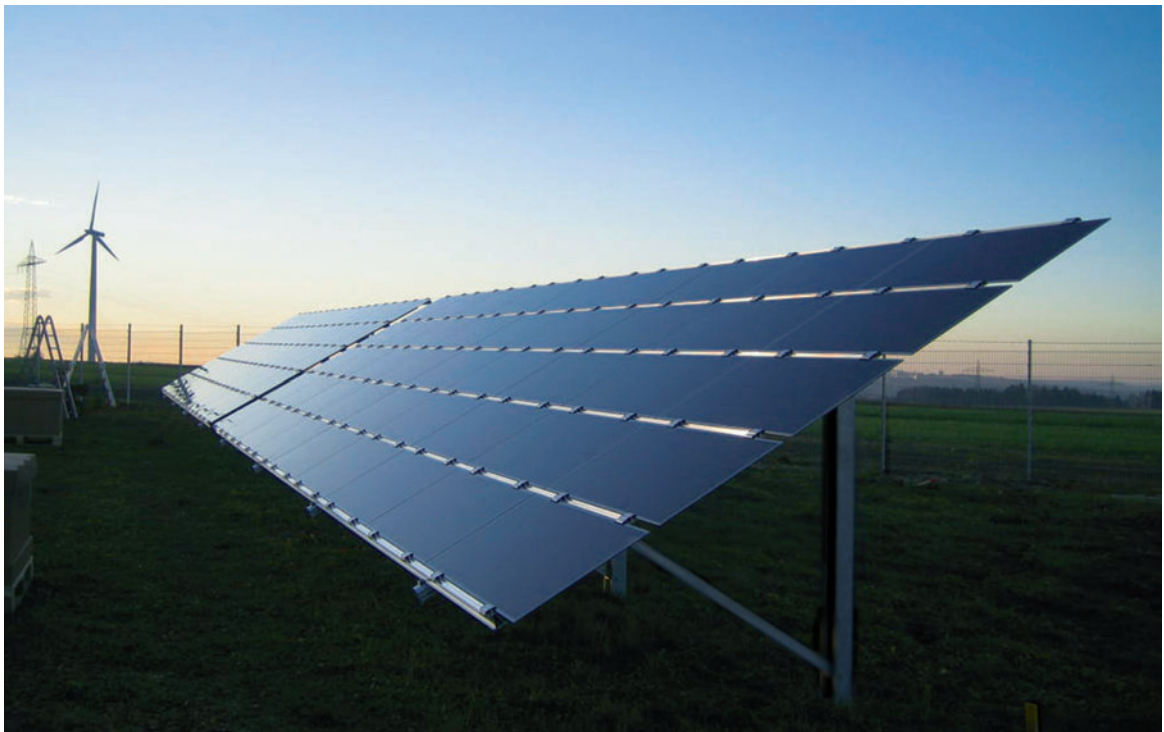
Haunsfeld - open-area solar park of thin-film modules with a total capacity of 1.67 MWp
