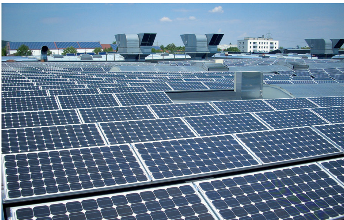
Keiper Recaro - rooftop solar power plant of mono-crystalline modules with a total capacity of 609 kWp
