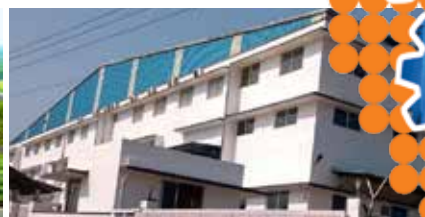
Khopoli, Maharashtra Installed capacity of 80,000 MTPA
