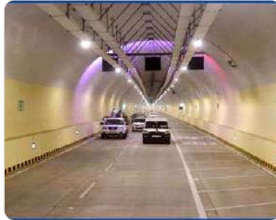
Mumbai Coastal Road Project twin Tunnel Lighting with Intelligent controls
