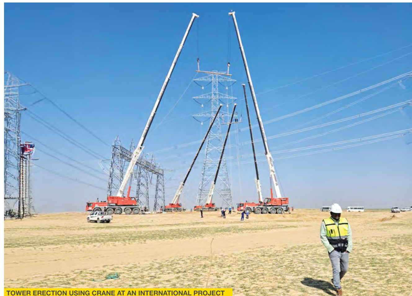
TOWER ERECTION USING CRANE AT AN INTERNATIONAL PROJECT
