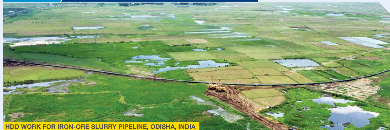
HDD WORK FOR IRON-ORE SLURRY PIPELINE, ODISHA, INDIA
