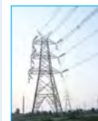
400KV D/C Dhalkebar - Bathnaha TL, Nepal
