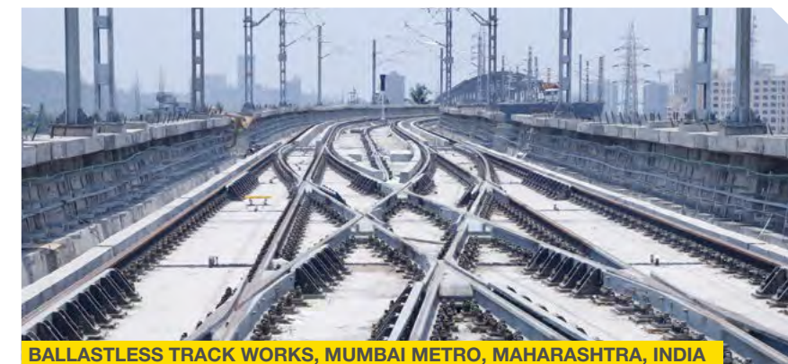
BALLASTLESS TRACK WORKS, MUMBAI METRO, MAHARASHTRA, INDIA
