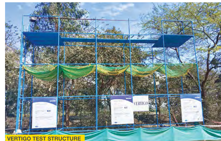
VERTIGO TEST STRUCTURE
