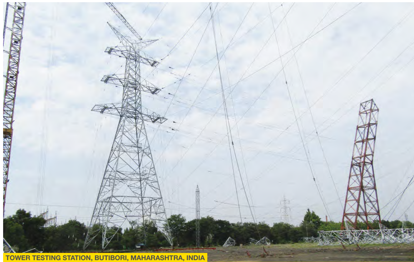
TOWER TESTING STATION, BUTIBORI, MAHARASHTRA, INDIA
