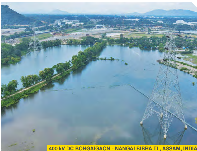
400 kV DC BONGAIGAON - NANGALBIBRA TL, ASSAM, INDIA
