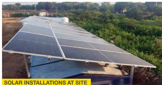
SOLAR INSTALLATIONS AT SITE
