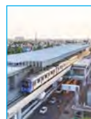
Elevated Metro Rail Project, Chennai
