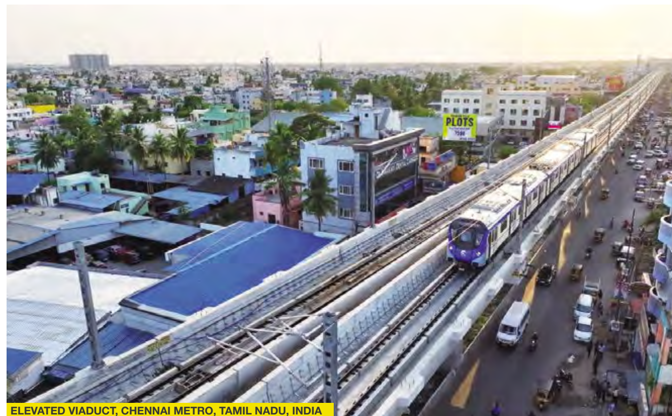
ELEVATED VIADUCT, CHENNAI METRO, TAMIL NADU, INDIA
