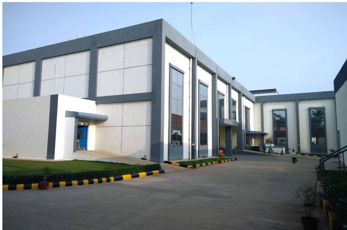
CP-I plant at Suthukeny, Puducherry
