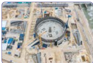
NHT-CCR Reforming Unit at Arzew Refinery
