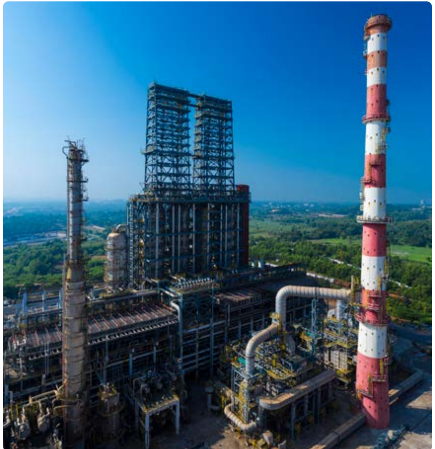
Delayed Coker Unit (DCU) at Mangalore Refinery
