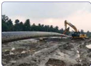
Dobhi-Durgapur-Haldia Pipeline Project
