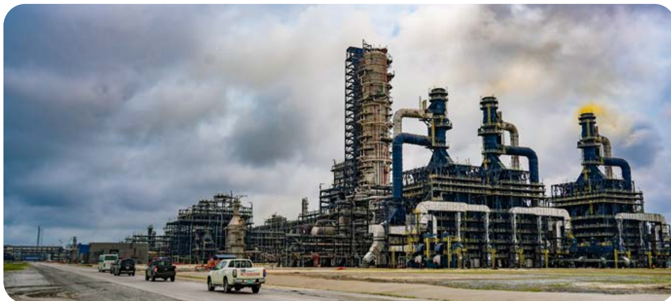
Dangote Refinery Project, Nigeria
