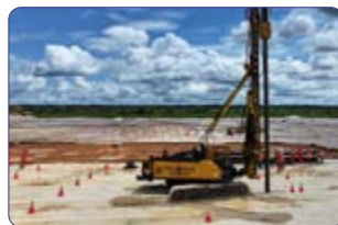
Integrated NGL Plant and 300 MW CCGT Power Plant Project
