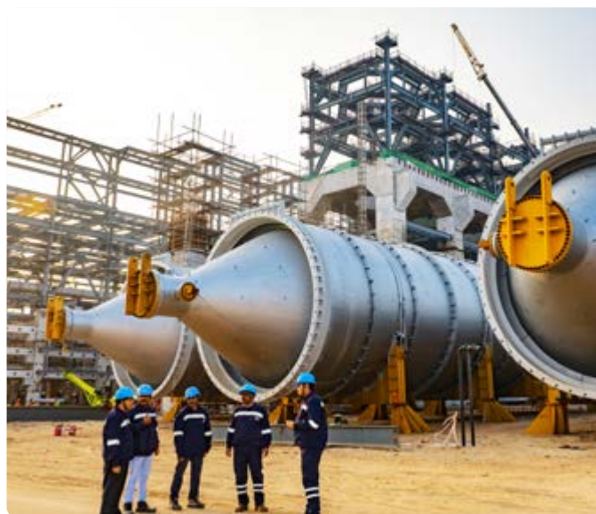
Rajasthan Refinery project
