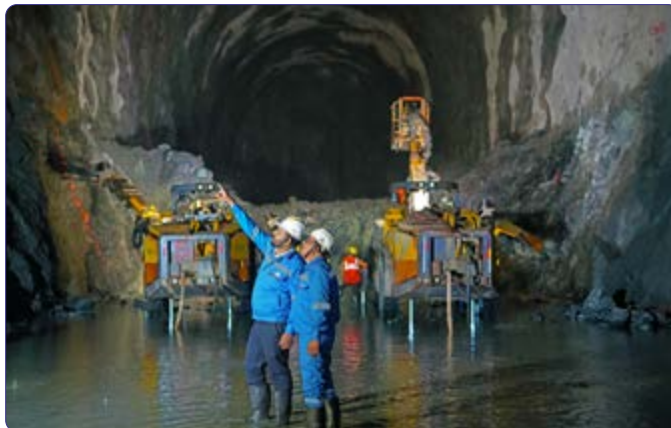
LPG Cavern Project, Mangalore
