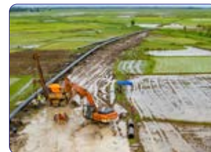
Upgradation of facilities for Numaligarh-Siliguri Pipeline
