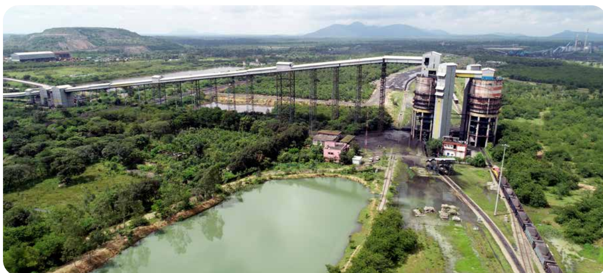
First Mile Connectivity project at SECL Dipka
