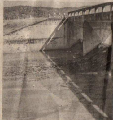
Dead water storage refers to the water in a dam's outlet and can only be pumped out
