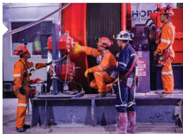
Deepening of the San Carlos shaft
