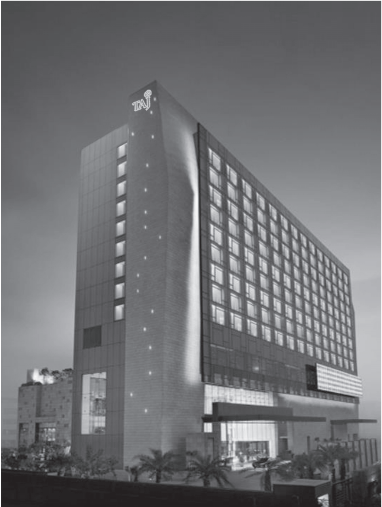
Company's Hotel Project- "TAJ CITY CENTRE - GURUGRAM" located at Plot No. 1, Sector 44, Gurugram, Haryana
