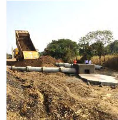
Village infra development
