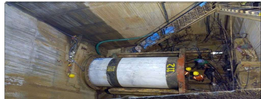
VMSS – Micro Tunneling Vadodara
