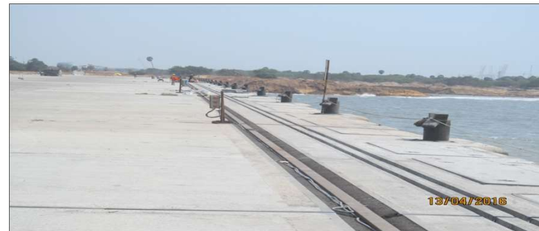
Ennore container terminal, Chennai
