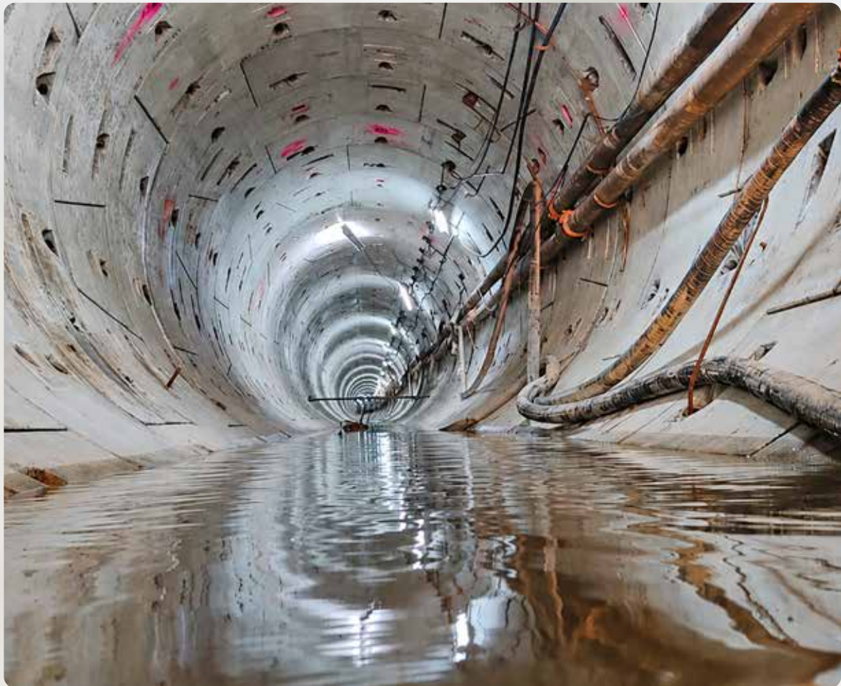
▲ MCGM Micro-tunnelling Project in Maharashtra
