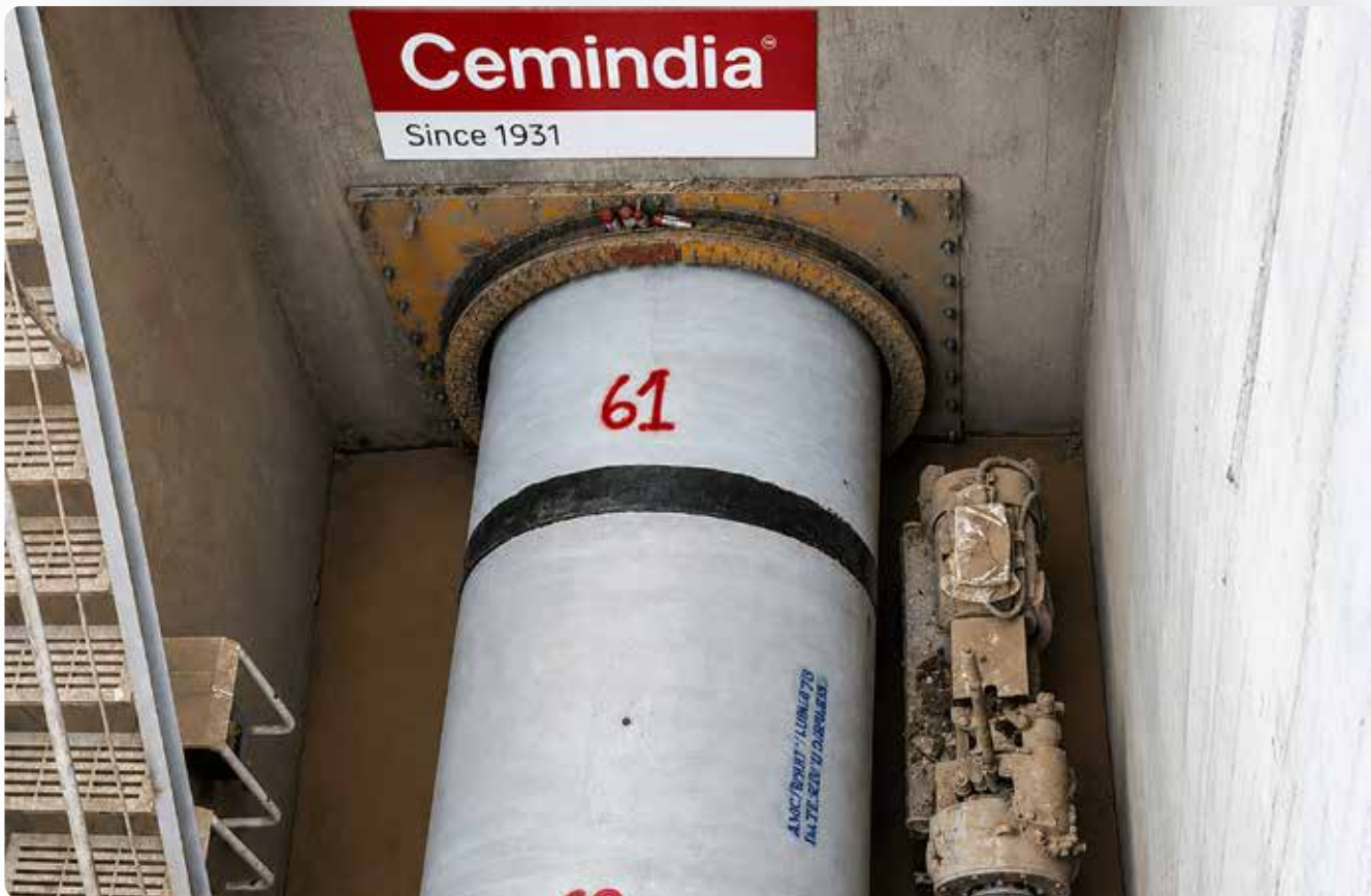
▲ Ahmedabad Micro-tunnelling Project in Gujarat
