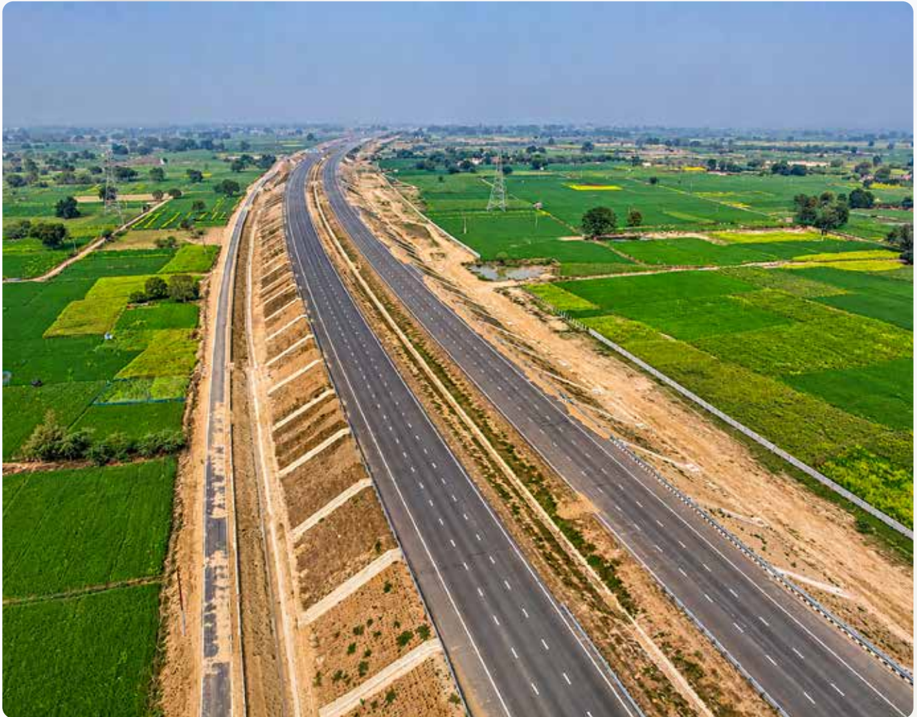
▲ Ganga Expressway Road Project in Uttar Pradesh
