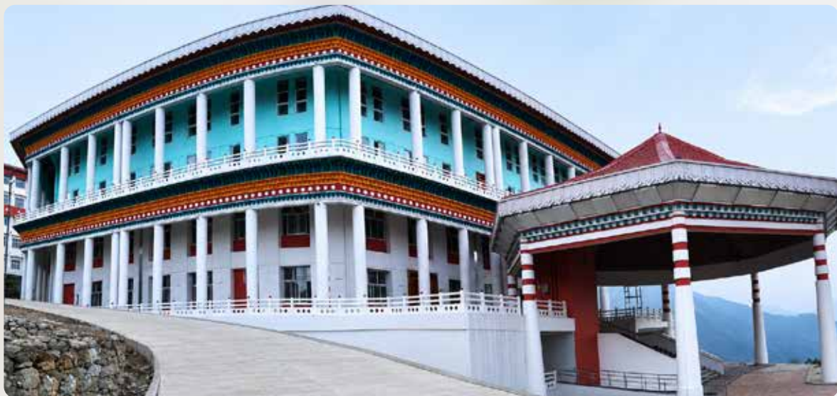
▲ University Building in Yangang, Sikkim
