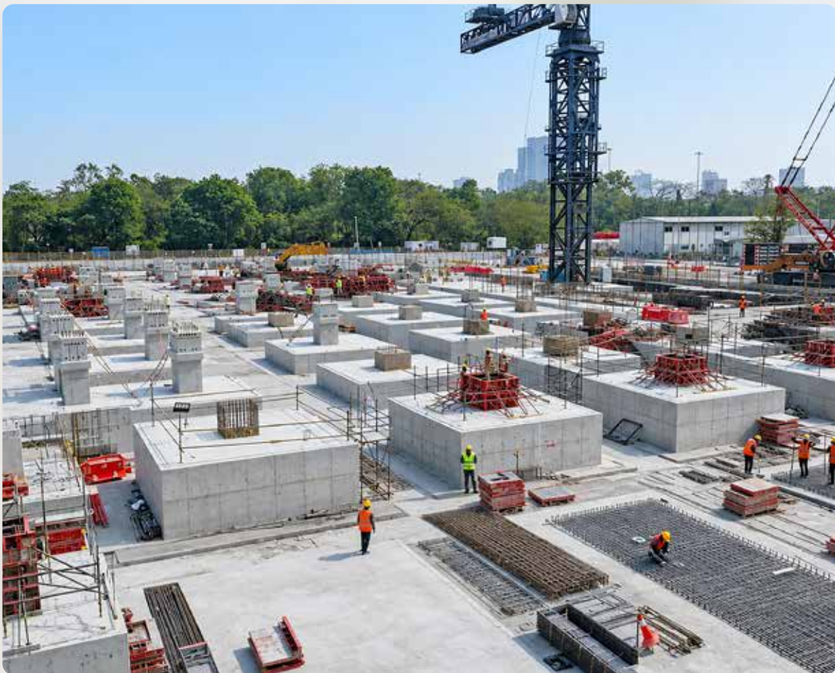
▲ Data Centre Building Under Construction in Maharashtra
