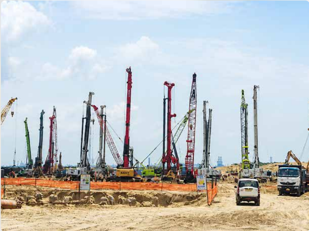
▲ Piling Work at JSW Utkal in Odisha
