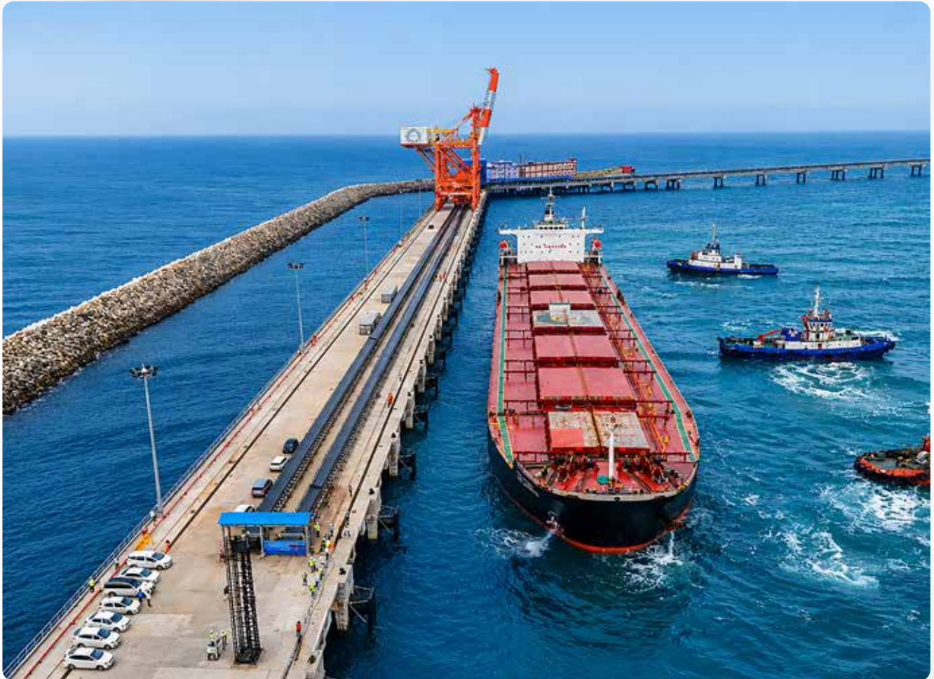
▲ Udangudi Marine Project in Tamil Nadu
