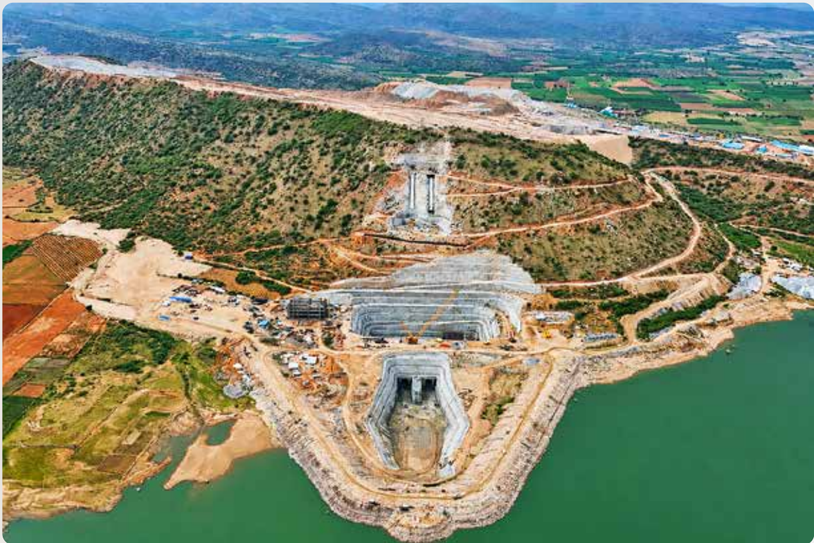
▲ Chitravathi Pumped Storage Project in Andhra Pradesh
