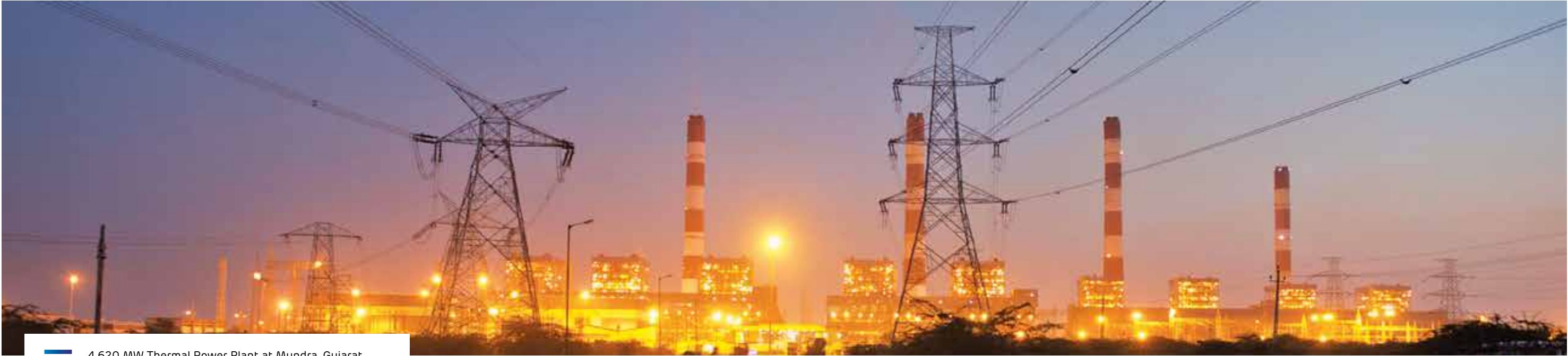
4,620 MW Thermal Power Plant at Mundra, Gujarat
