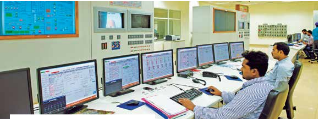
Thermal Power Plant at Tiroda, Maharashtra
