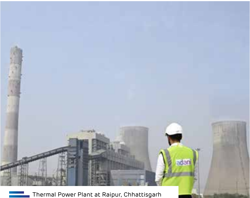
Thermal Power Plant at Raipur, Chhattisgarh
