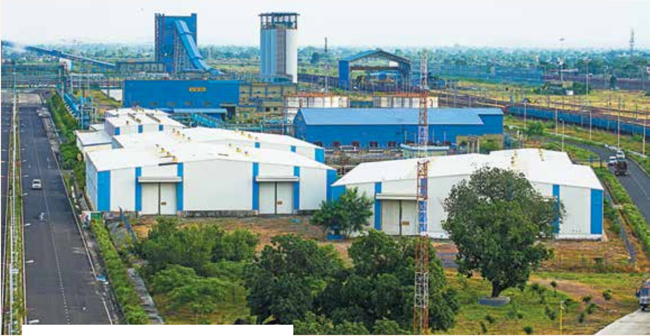
Thermal Power Plant at Kawai, Rajasthan
