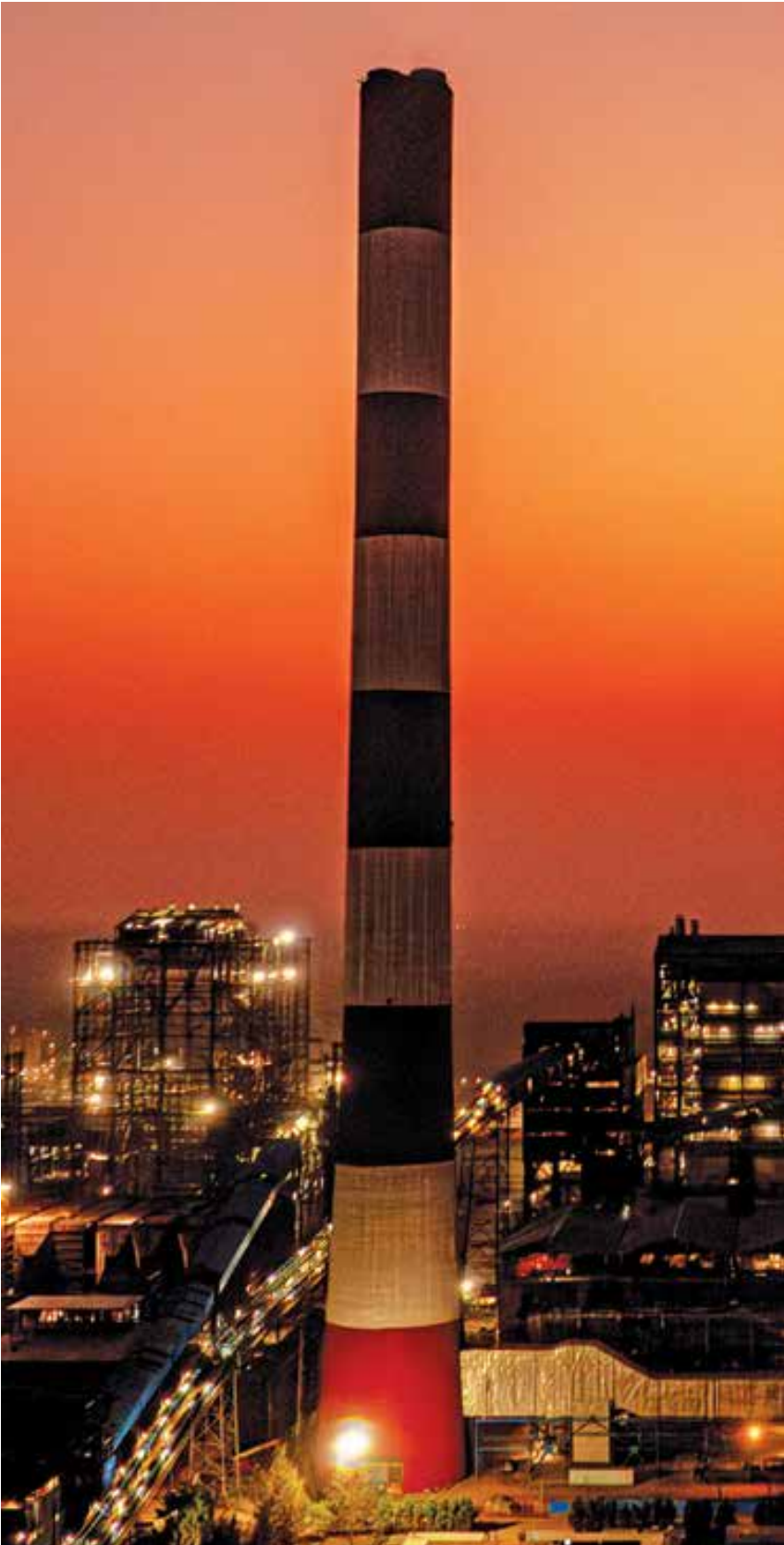
Thermal Power Plant at Raipur, Chhattisgarh
