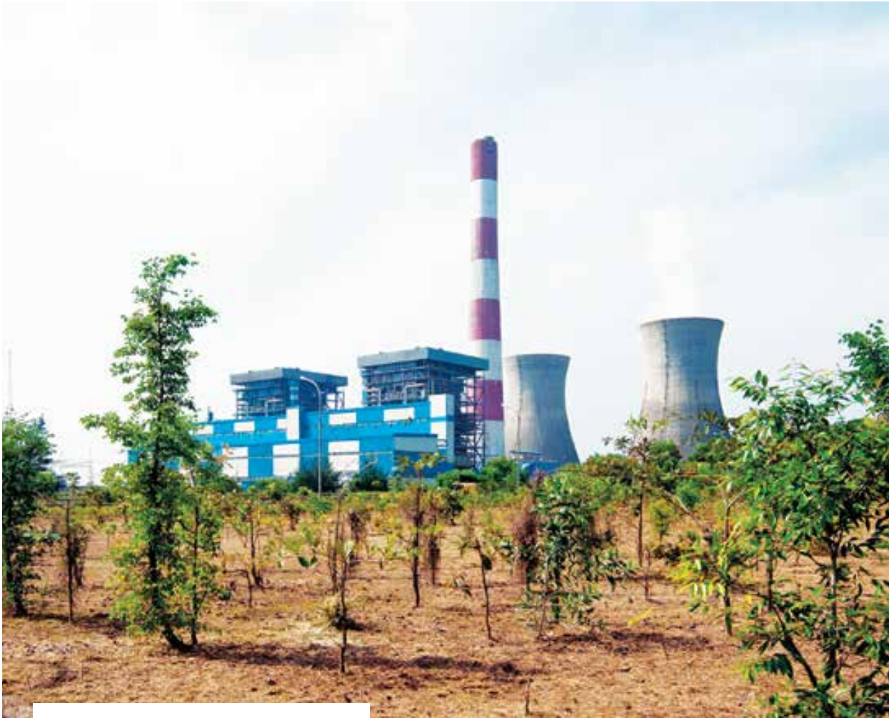
Power plant at Udupi, Karnataka
