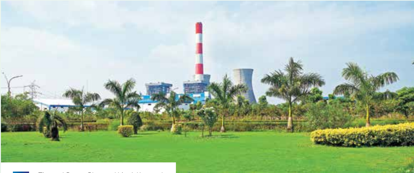
Thermal Power Plant at Udupi, Karnataka
