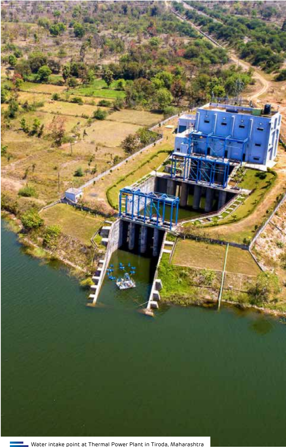
Water intake point at Thermal Power Plant in Tiroda, Maharashtra
