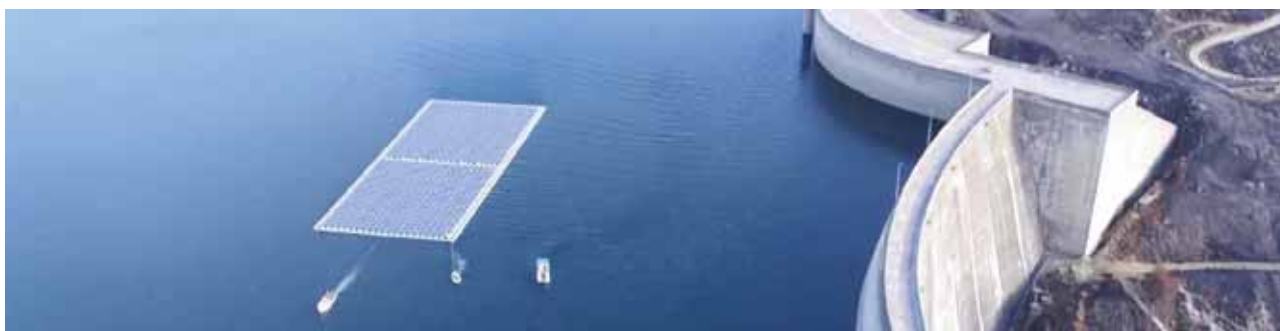
Alto Rabagão floating solar plant
