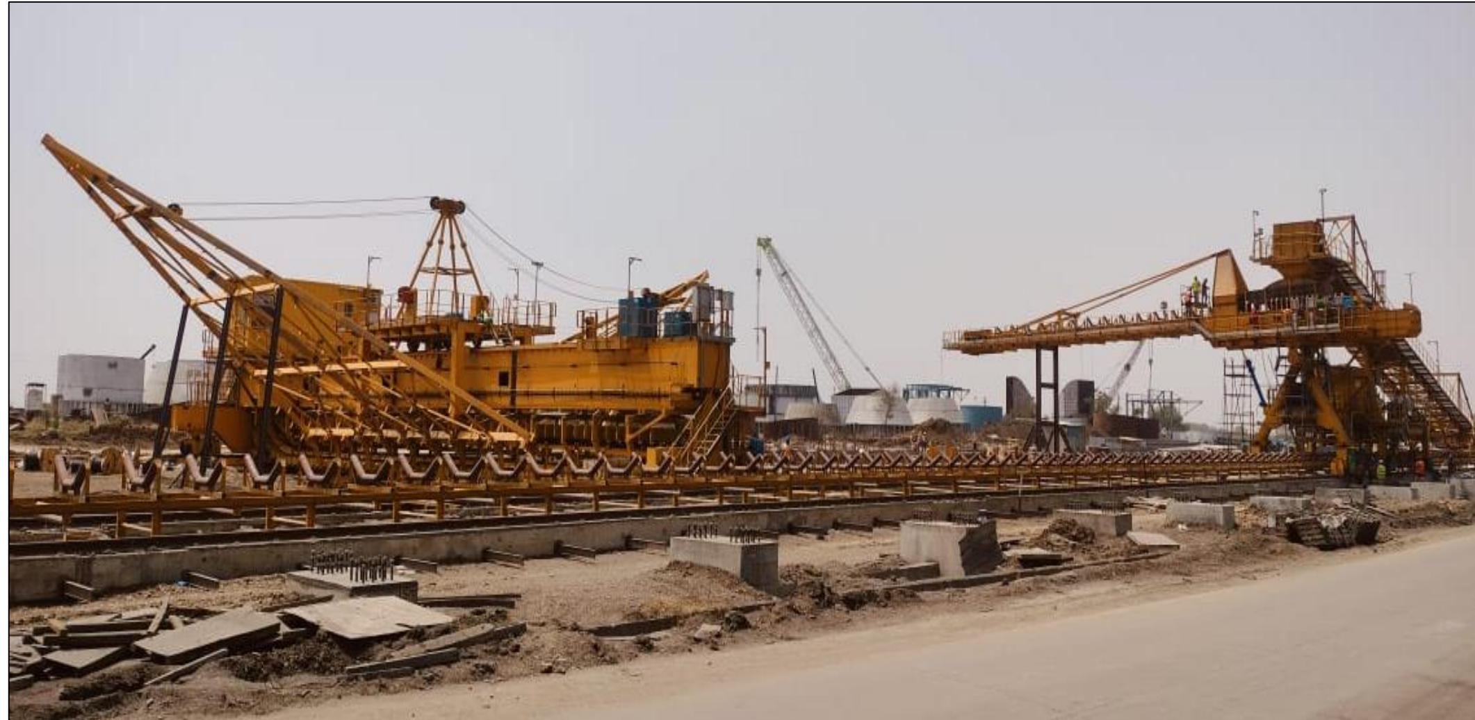
Limestone Stacker & Reclaimer
