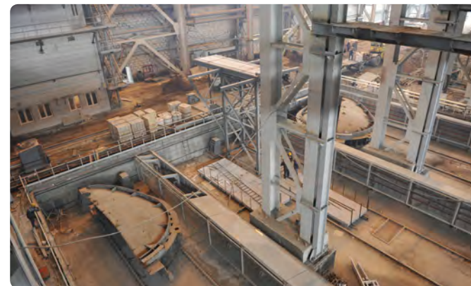
Construction of an electric arc furnace at TAGMET
