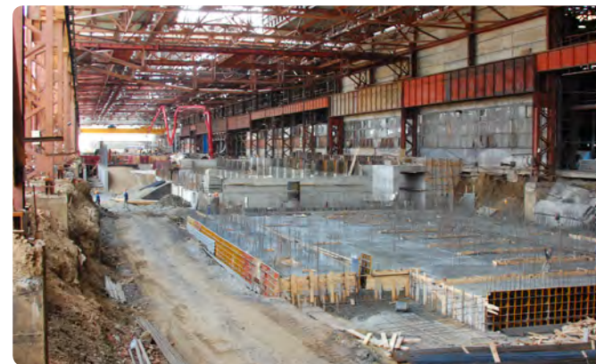
Construction of a continuous FQM pipe-rolling complex at Seversky Tube Works
