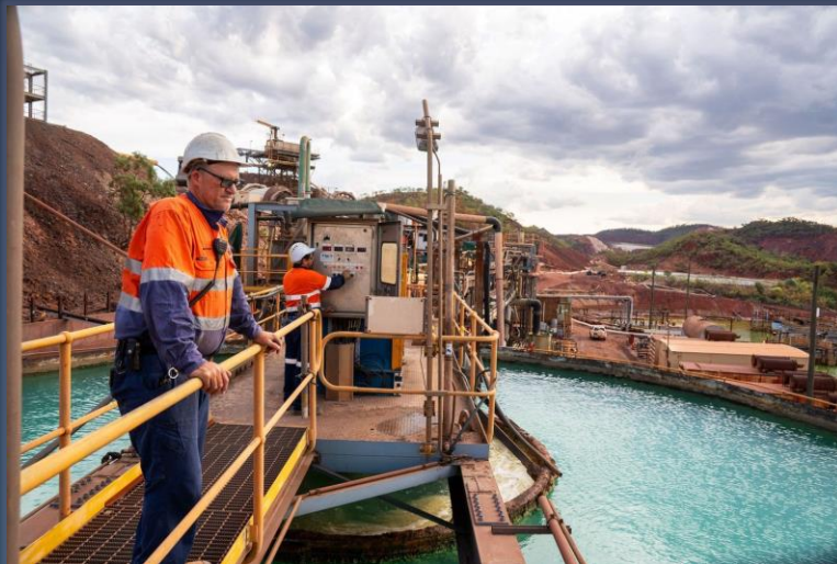
Processing plant & surface infrastructure
