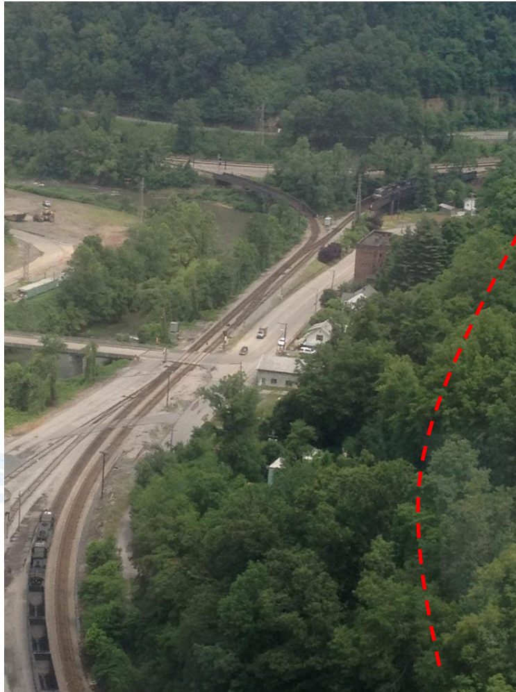
FIGURE 5 - RAIL AND THE TOWN OF IAEGER SHOWN ADJACENT TO THE APPROXIMATE SOUTHERN PROPERTY BOUNDARY
