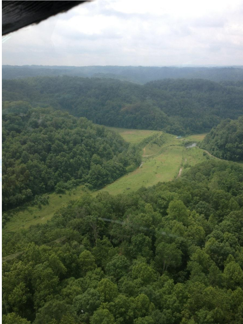
FIGURE 3 - VIEW OF EMMAUS PROPERTY AND OLD TAILINGS DAM
