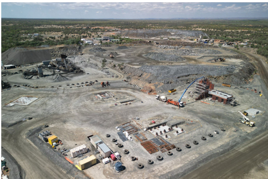
Photo: Current expansion work at Eloise. Mill raft concrete poured and backfilled (centre-left), and crusher suspended slab concrete pour (centre-right).
