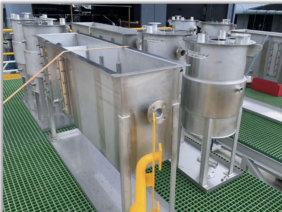
SX Module fabrication progress
