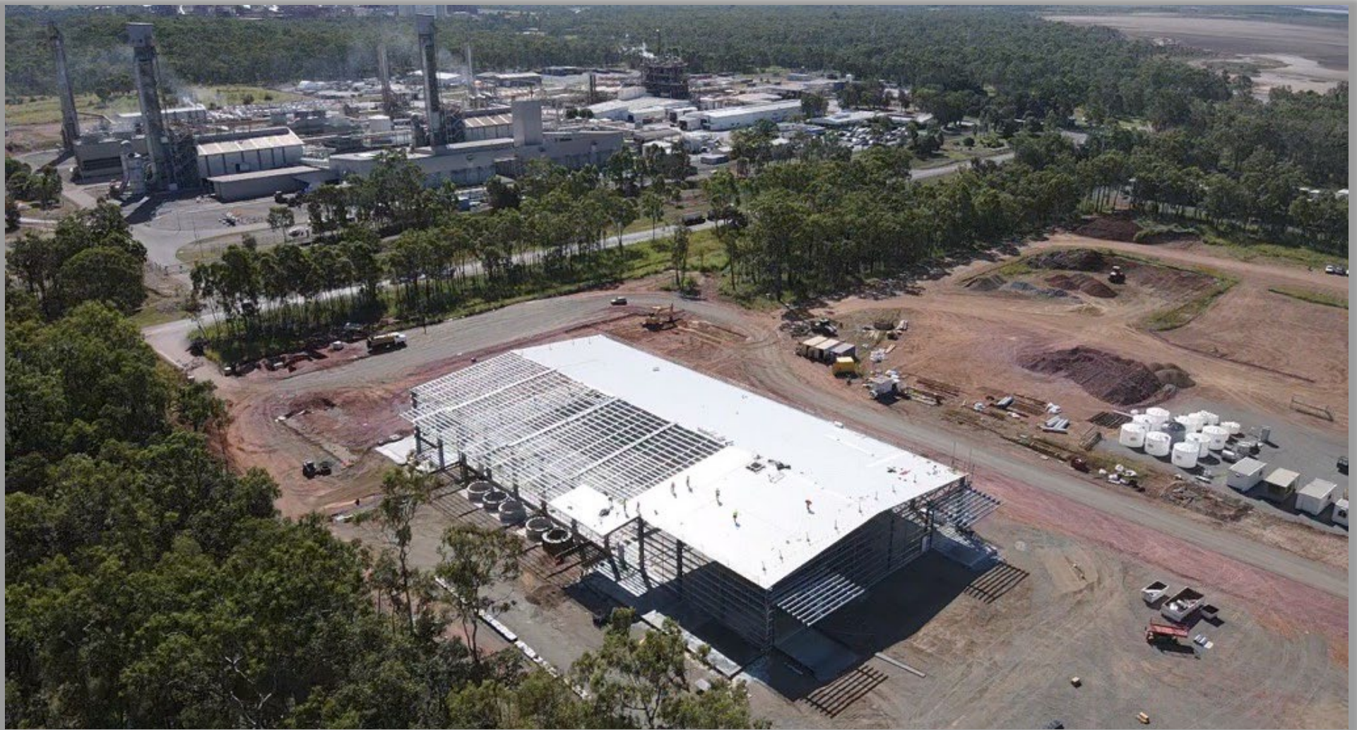
Cladding of the main PPF building is well advanced
