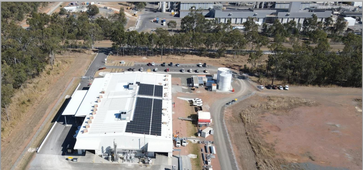
Stage 1 PPF – showing rooftop solar installation
