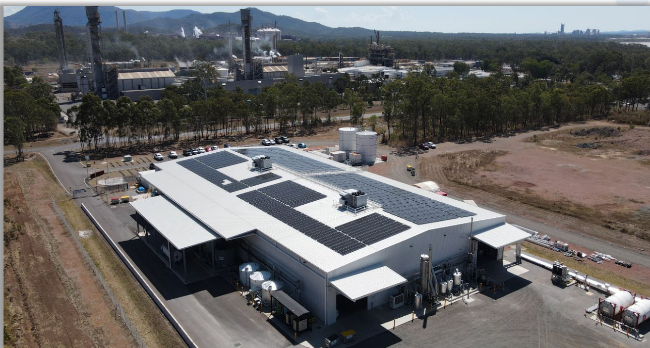
Stage 1 PPF – showing completed rooftop solar installation
