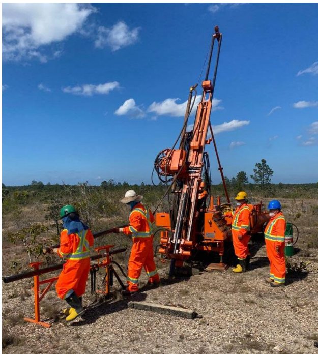
Diamond Drill Rig
