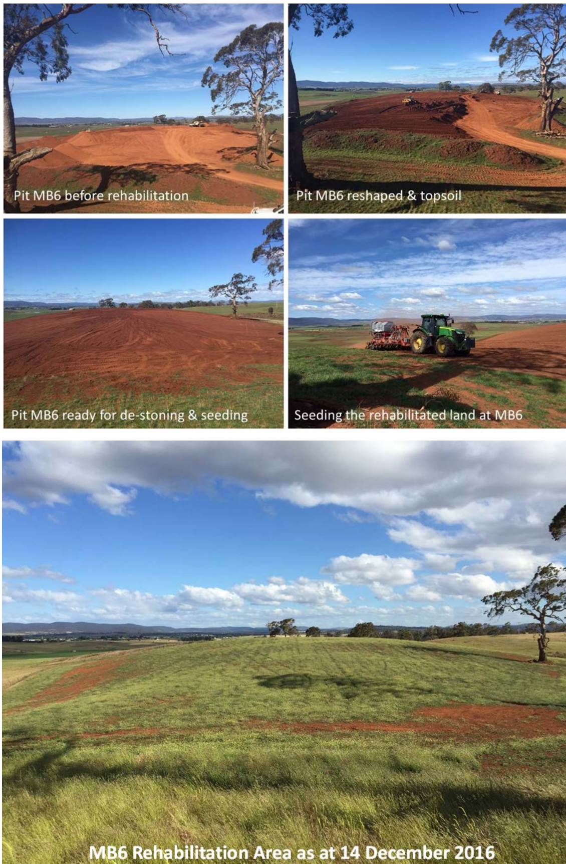
Figure 4: photographic record of rehabilitation processes, with Pit MB6 as the case study
