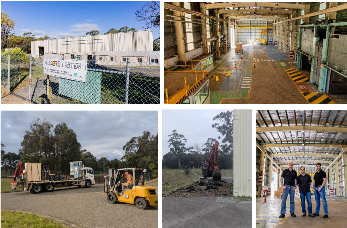
Figure 3: Construction activities and equipment delivery at the ALCORE Technology Centre
