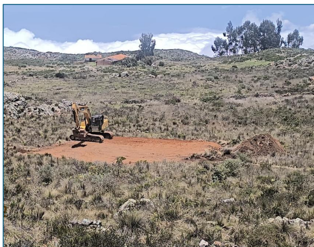
Image 3: Drill pads at Flint
