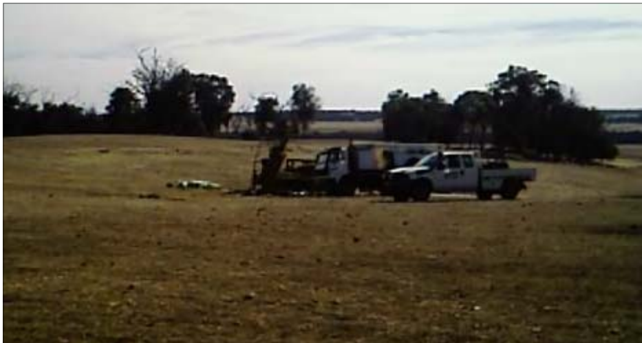
Exploration Drilling at Katanning
