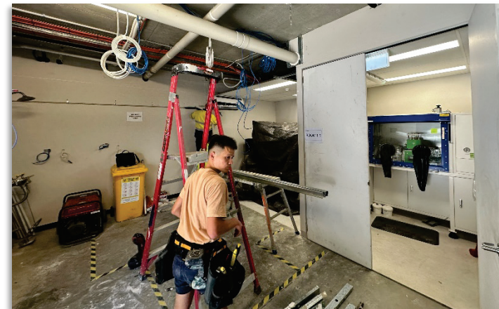
Above: Expansion to battery testing laboratory in progress
