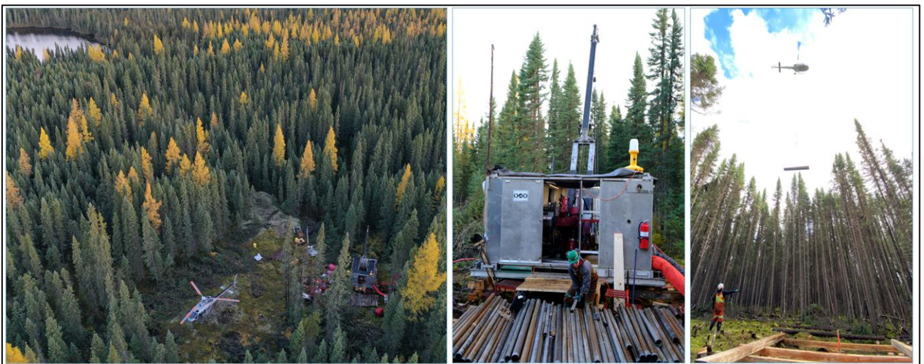
Figure 7 – Drill Pad Setup at Ardiden's Kasagiminnis Gold Deposit
