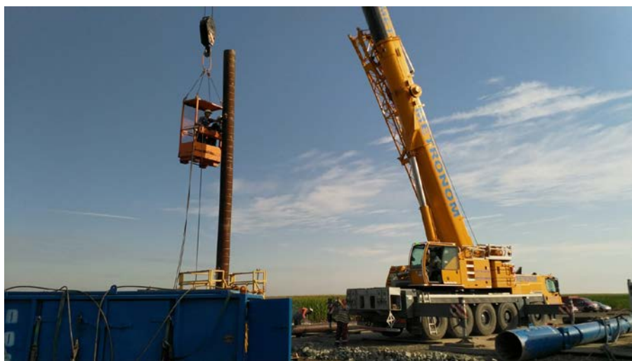
Ilecea Mica – 1 Well Conductor Casing Installation
