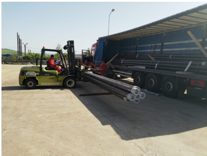
Ilecea Mica – 1 Well Casing delivery.
