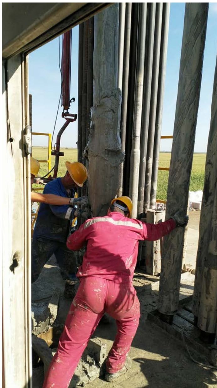
Tacrom Futura 6 Rig Floor – Pulling out of 12 ½" hole
