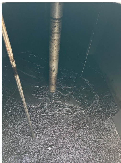
Figure 2: Anshof-3 crude oil (open tank) produced through the new Permanent Production Facility (PPF)
