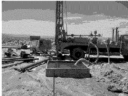
Drilling rig and prime tank
