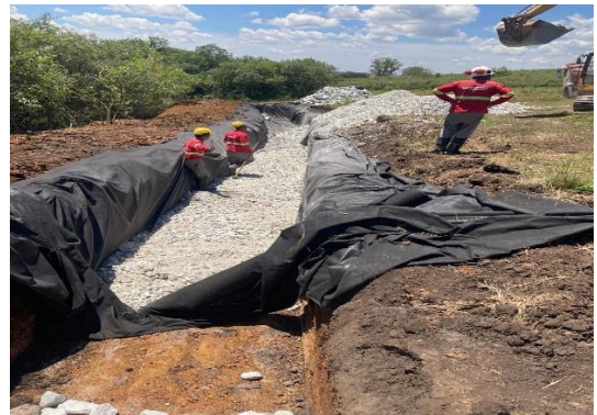
Image 2: Drainage to sump advancement
