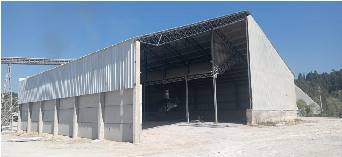
Photo 1 Run of Mine Storage complete
