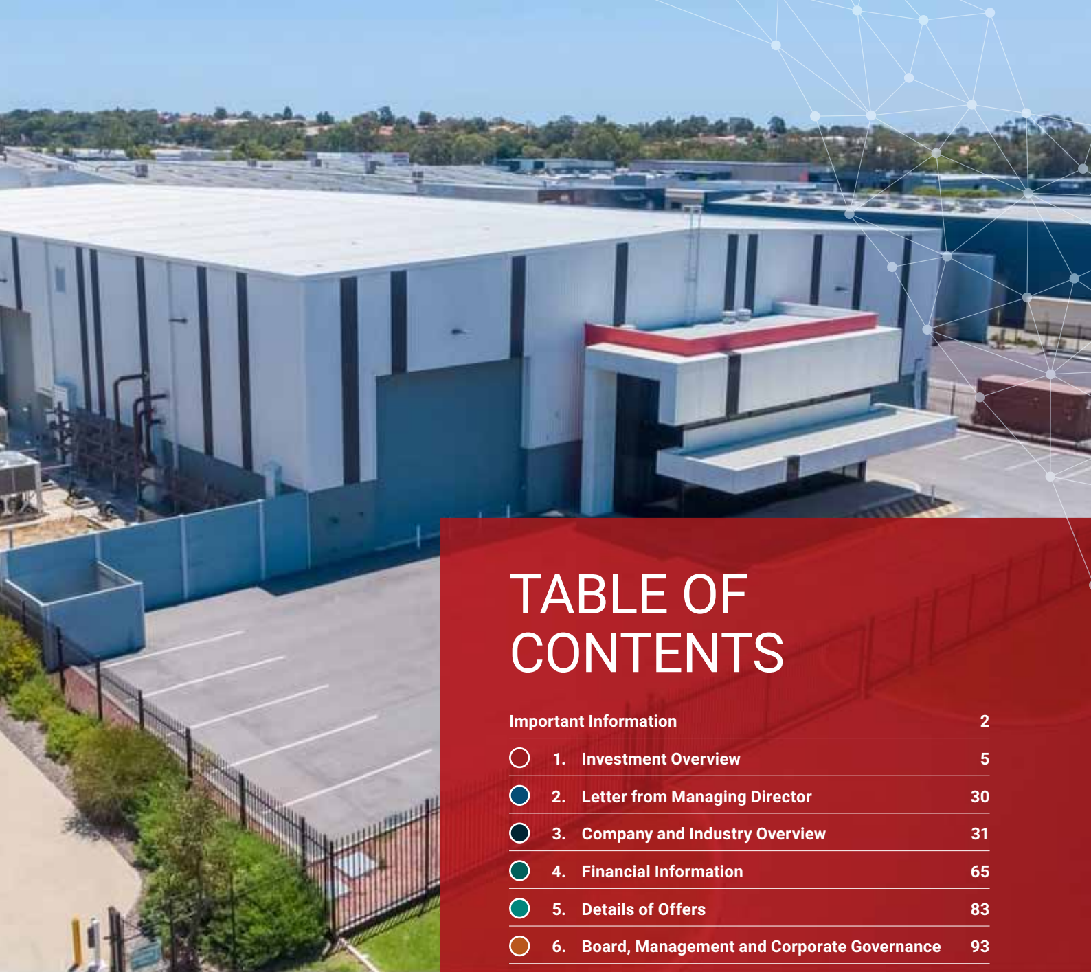
Image showing the new Bibra Lake Data Centre facility
