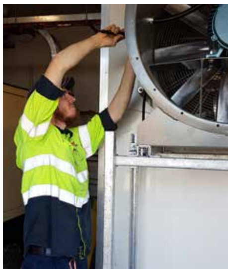
Electrical technician installing the modular data centre cooling fans
