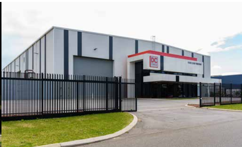
New signage installed at DC Two's Bibra Lake data centre
