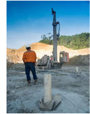
Drill and Blast
