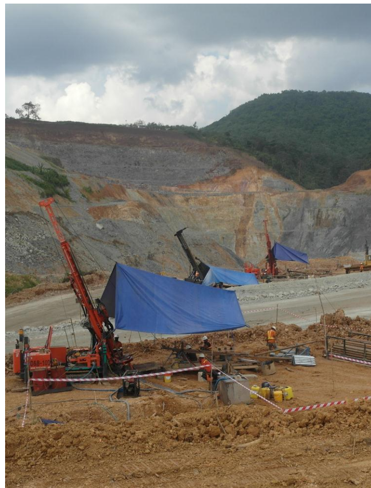
Diamond drilling, Permata resource drillout
