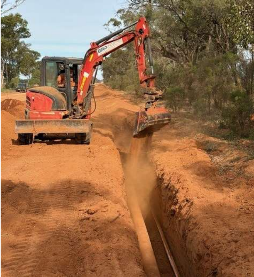
Figure 1: Trenching activities on the services corridor
