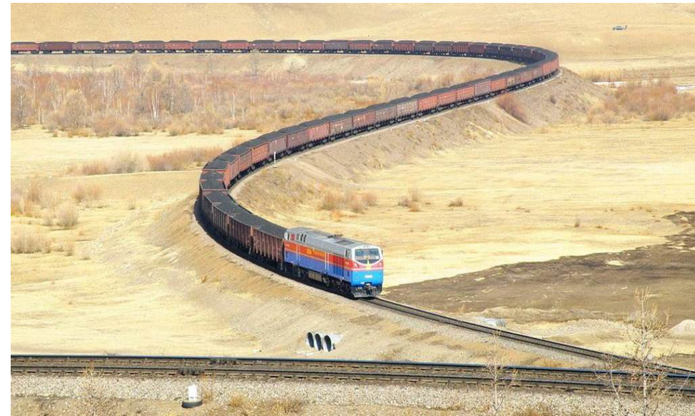
Trans-Mongolian Railway, coal from Baganuur coal mine
