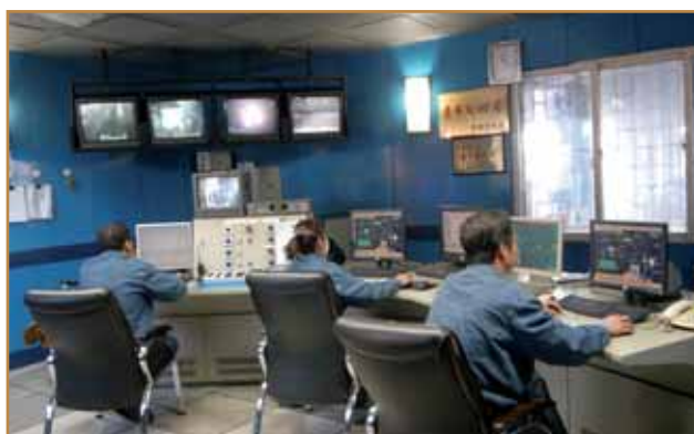
ISA Smelter Control Room at Kunming, China
