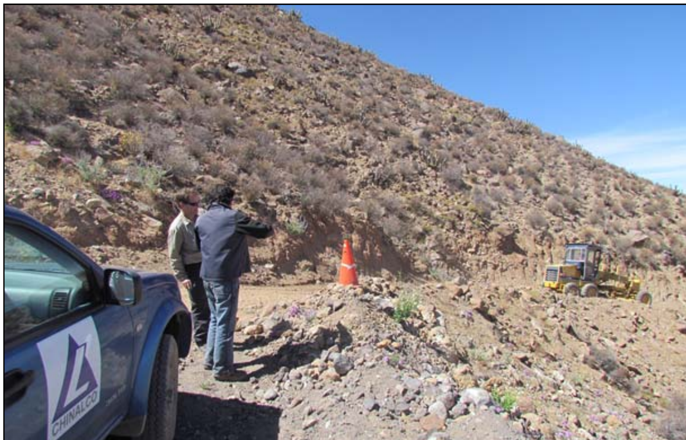
Road cleaning to the Candelabro Prospect – October 2011.
