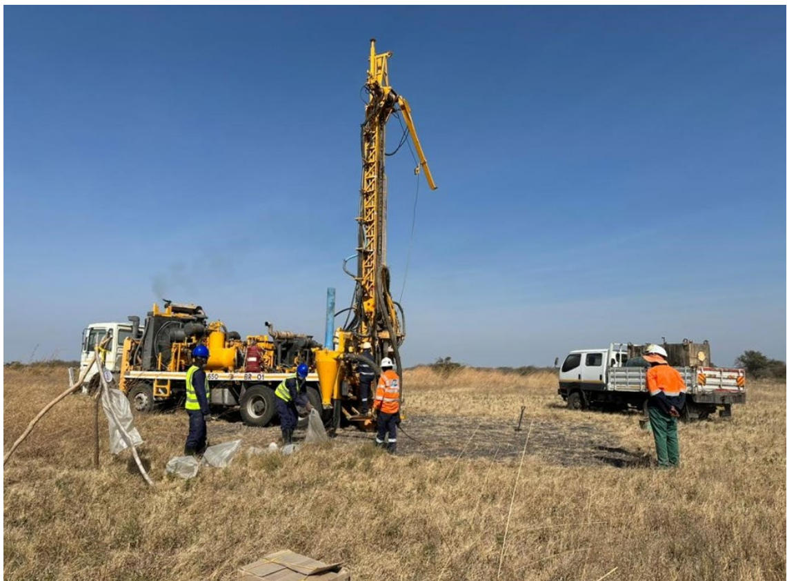
Figure 3 – Air core drilling rig at Itigi
