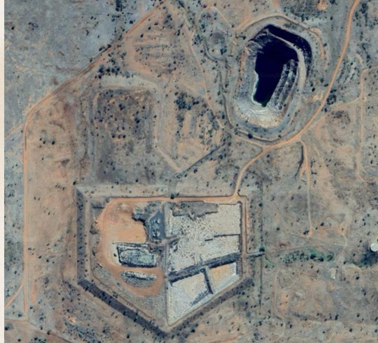
TICK HILL MINE AND TAILINGS STORAGE
