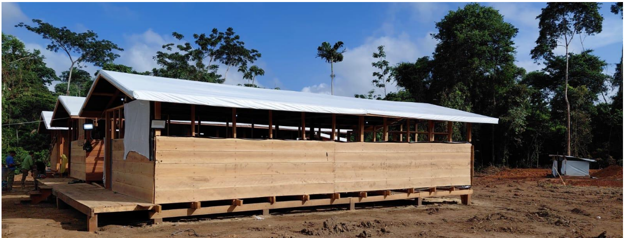
Figure 12: SOKO trench camp progress in early February.
