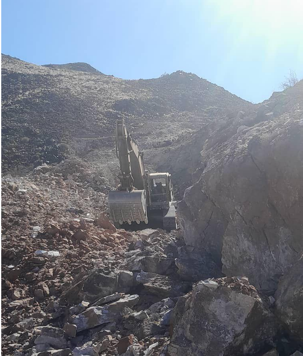
Figure 2 – Road construction in progress
