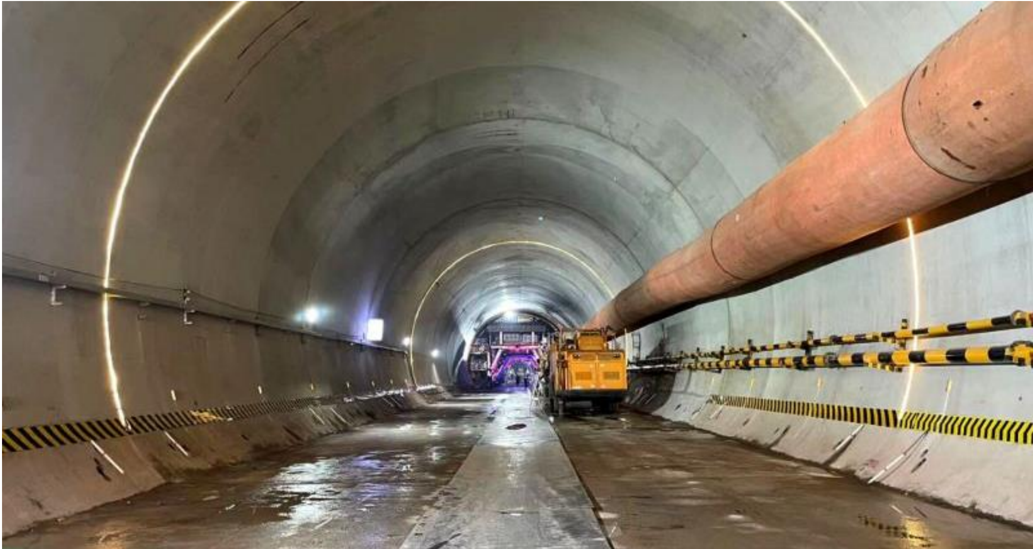
Kindia railway tunnel part of the multi-user rail network linking Simandou with the MoréBaya Port.
